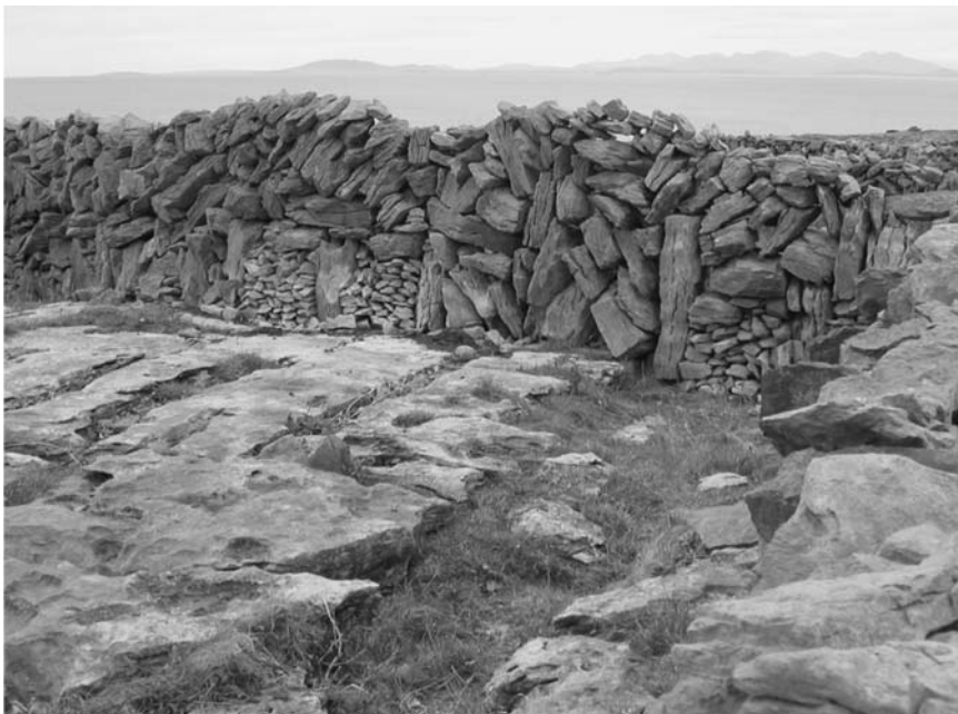
Figure 3 Older-built walls found 'back west'
