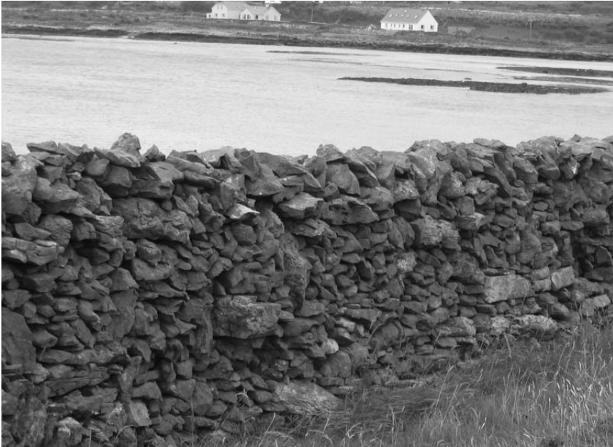
Figure 4 The newer walls found nearer the main village
